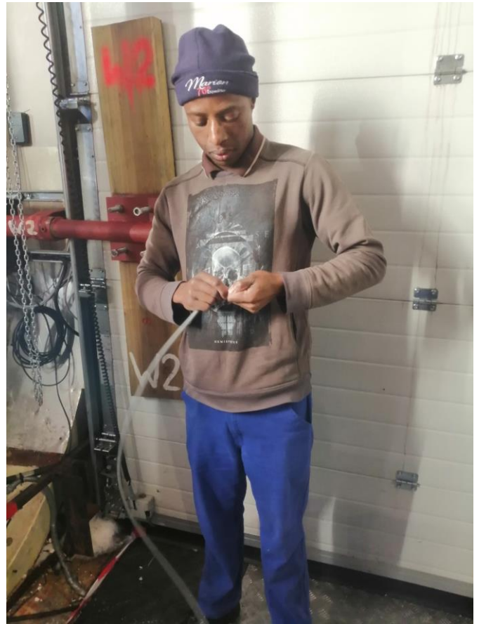
Hard at work with Fibre cables
