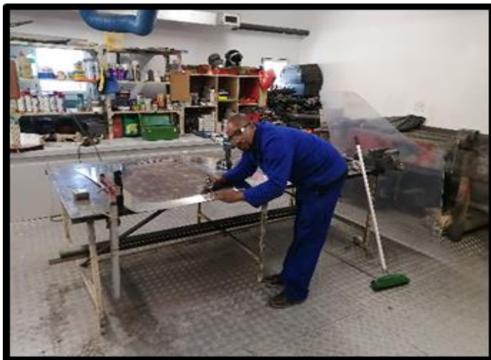
Thulz marking on the door frame where final trimming must be done
