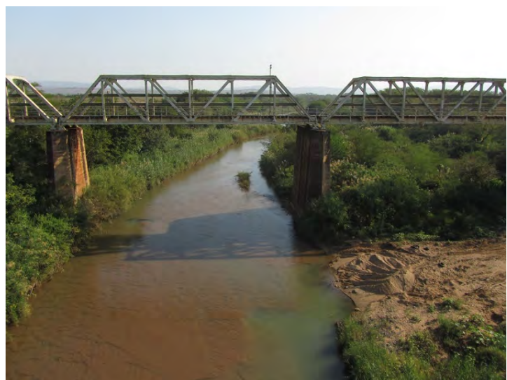
Mkuse railway bridge still standing
